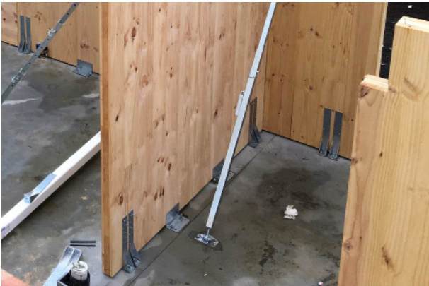
Angle brackets for tensile and shear connection.
