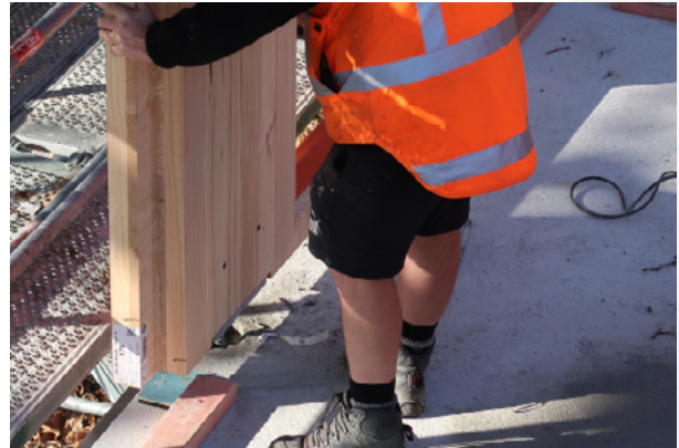
Prior checking avoids delays and minimises crane time.
