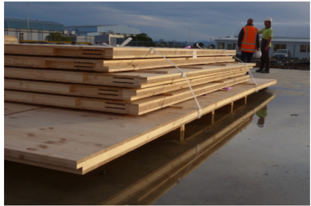
Insufficient end support may cause panel deformation.
