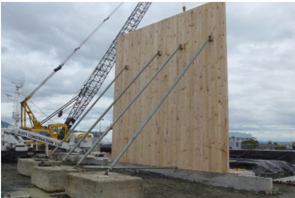
Walls are propped from the Industrial Appearance Grade side.
