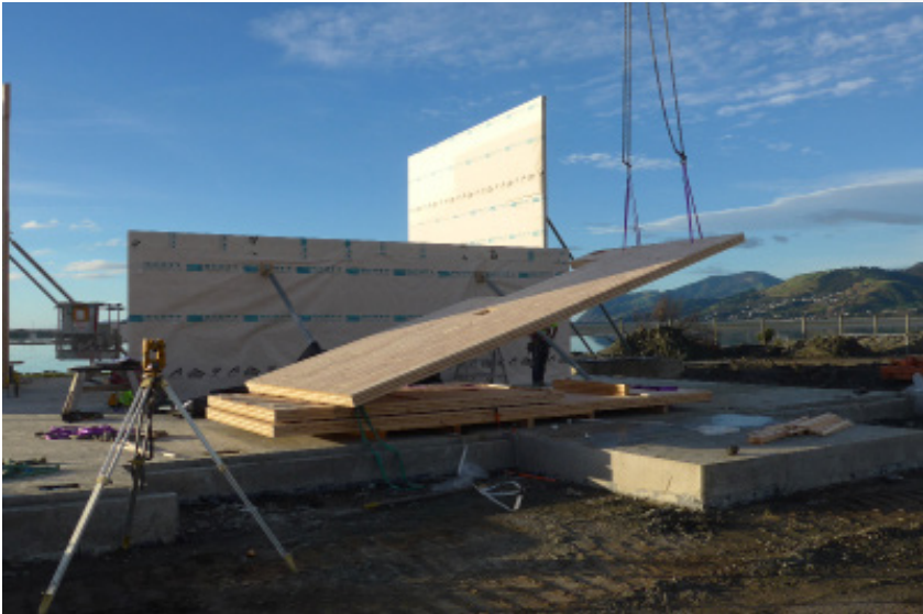
Lifting a wall panel off the stack.
