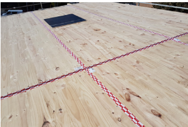
Taped joints to floor panels.
