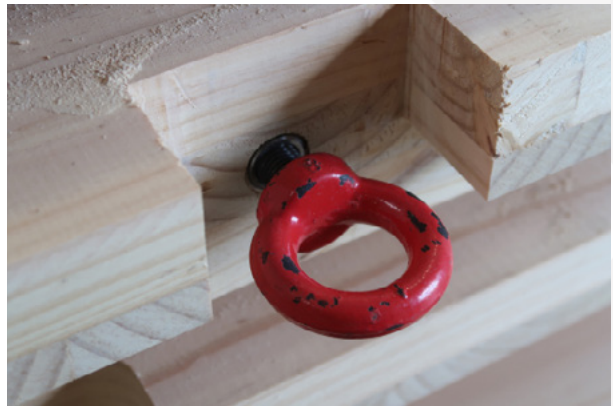
The sacrificial Rampa insert accepts a threaded lifting eye.
