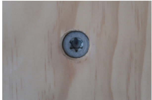
Countersinking the timber surface will prevent crushing around the screw head.
