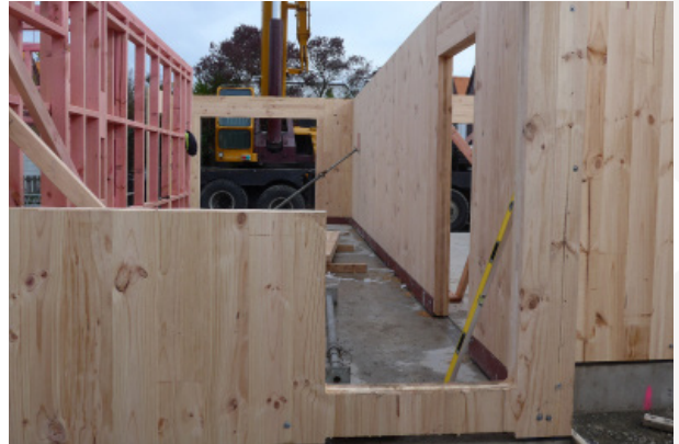
The door threshold will be cut out after installation.
