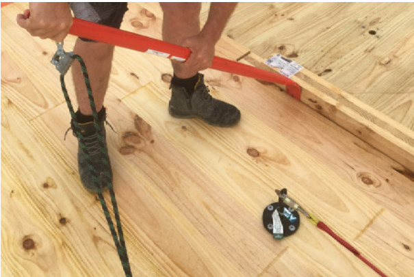
Bar and Xtraint safety anchor.
