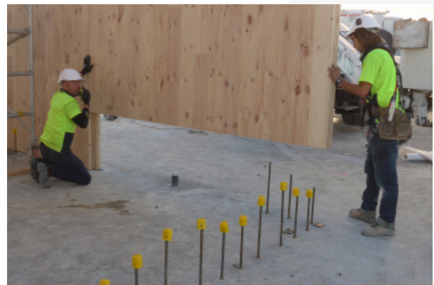
Sequential placement of wall panels.
