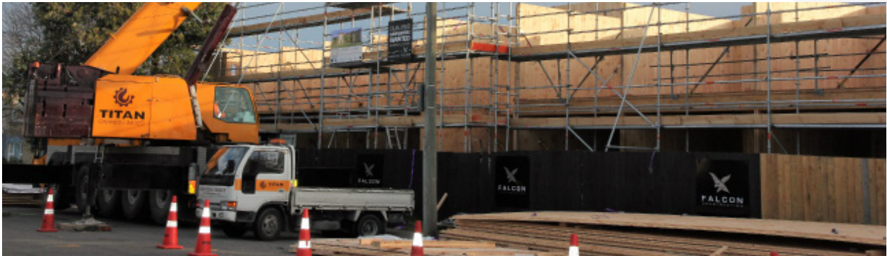
Partial road closure at a restricted construction site.
