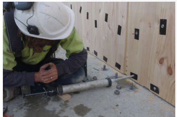
Pumping in epoxy adhesive to the encased dowels.
