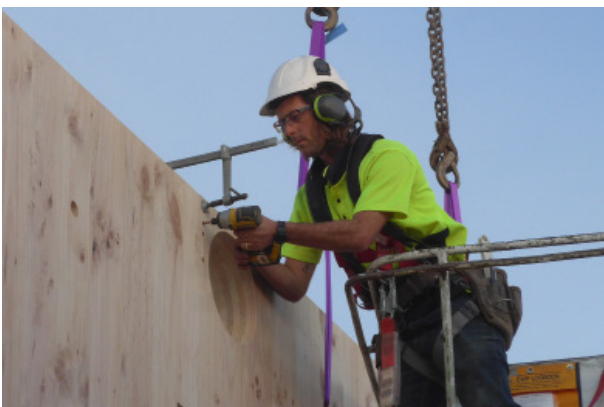
Clamping and screwing a wall panel joint at the top edge.
