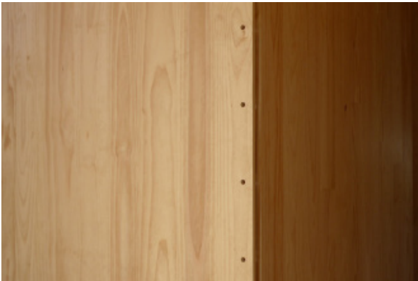
Screws neatly set out with heads counterbored to receive timber plugs.
