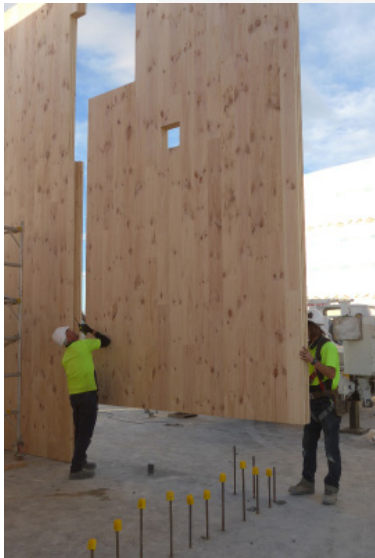
Lowering a panel into place.
