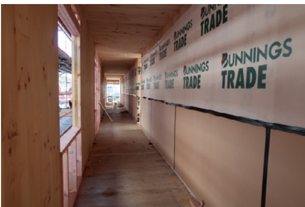
Use of fibreboard sheets to protect Natural Appearance Grade panels in high traffic areas.
