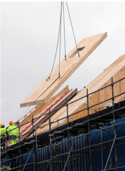
Lifting an inclined roof panel into position.
