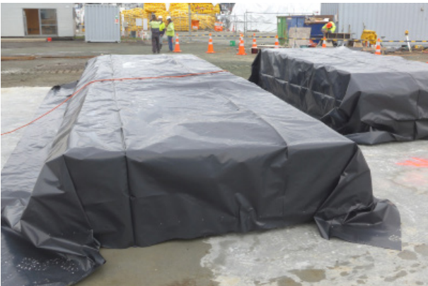
Panels must be well covered until needed for assembly.
