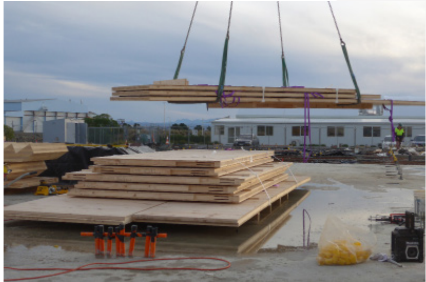
Craning a pack to temporary storage location.
