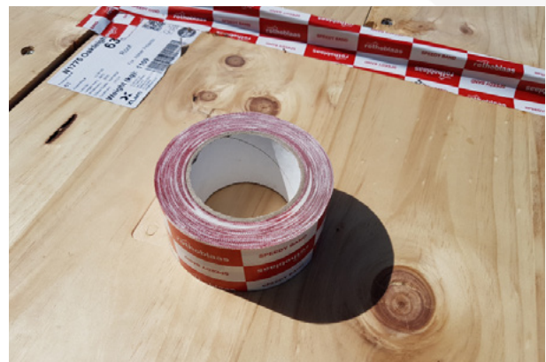
All end grain exposed to weather during construction is taped.
