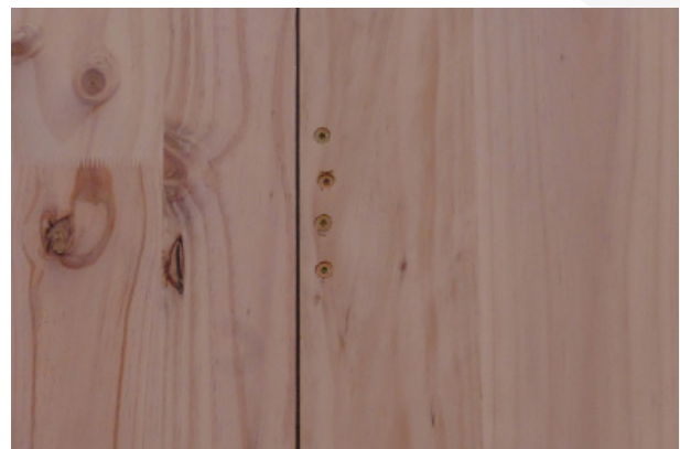
Partially threaded screws will draw a wall joint tight.
