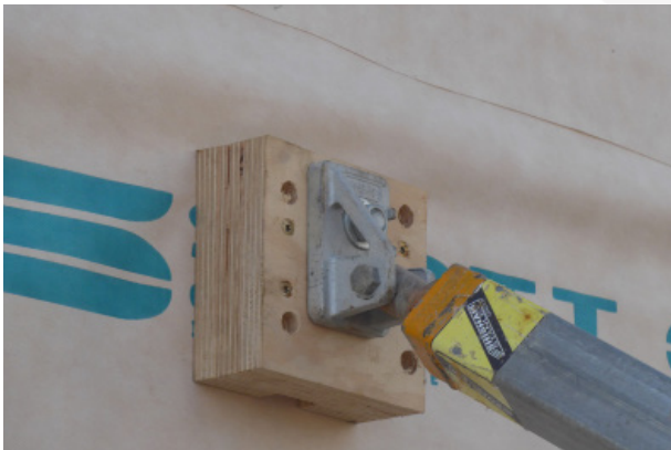
Prop connection with packing to a Natural Appearance Grade panel.
