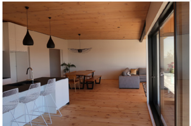
XLam Natural Appearance Grade panels showing a range of appearance quality.
