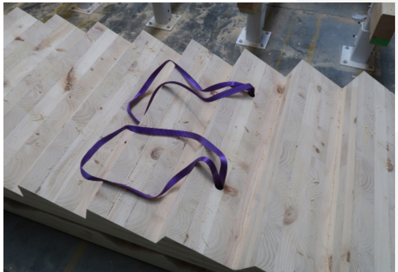
Centrally located lifting allows manual tilting of a suspended AirStair.
