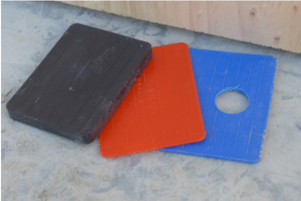
Graduated shims for base-levelling wall panels.
