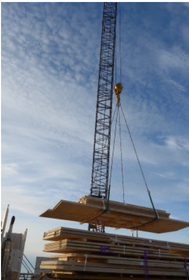
Panel packs craned off the delivery truck.
