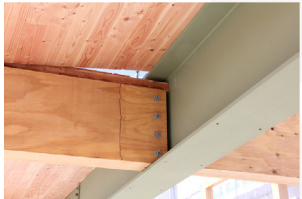
Hybrid structures need adequate tolerance for assembly.
