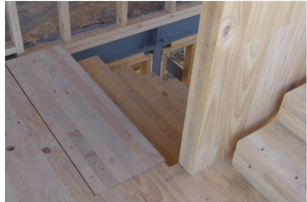
Screwed stair connections at the landings.
