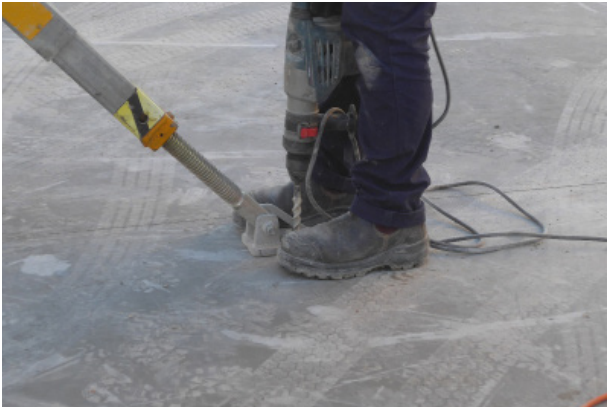
Prop connection to a concrete floor slab.
