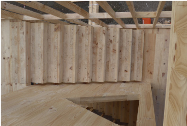
XLam AirStair spanning between landings and clear of side walls.
