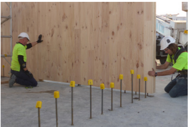
Factory-drilled panels fitted over steel dowels.
